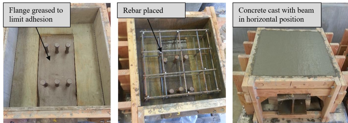
Figure 48 Placing concrete on steel beam sections by greasing steel flange, placing rebar, and casting concrete in horizontal position
