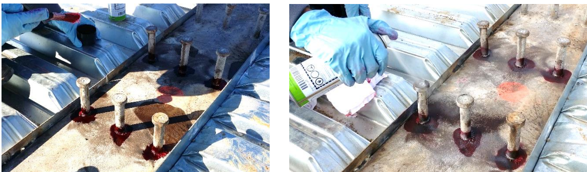
Figure 51 Shows penetrant applied and the developer being sprayed onto 6 shear studs
