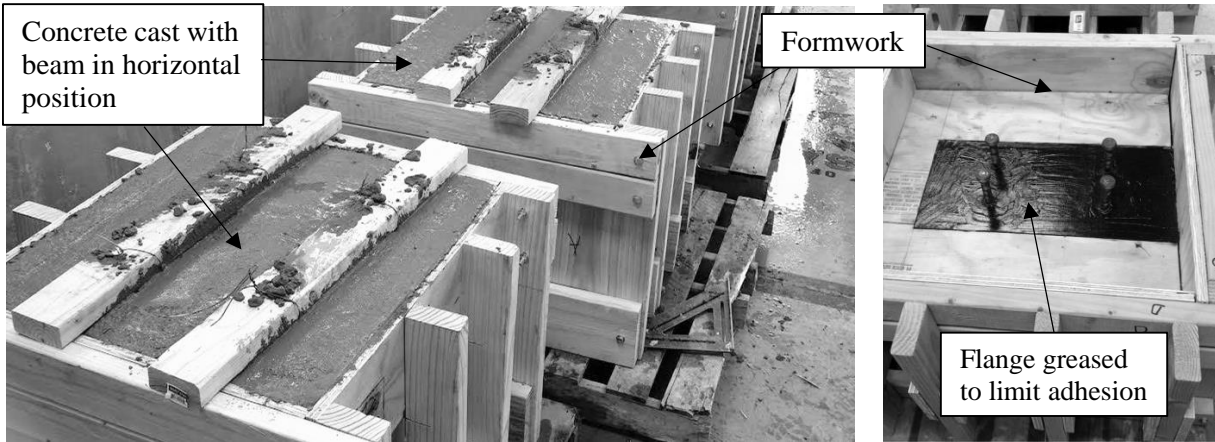
Figure 12 Casting of concrete slabs on double sided push-out specimens
